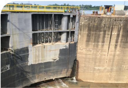
floating lock gate
